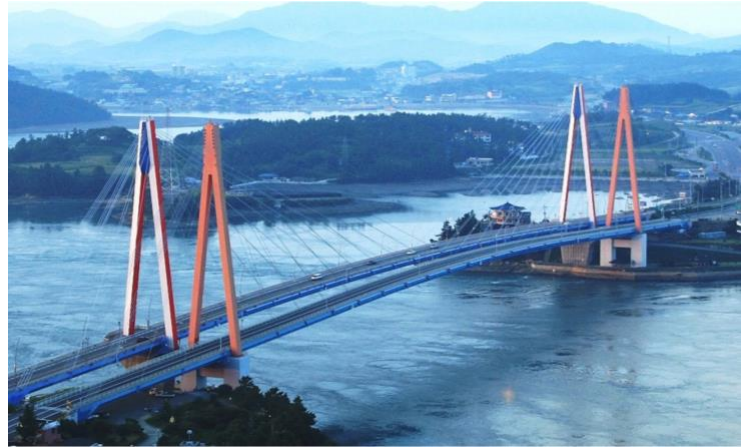
Wireless SHM, Jindo Bridge (South Korea). Link: goo.gl/NdB8iE
